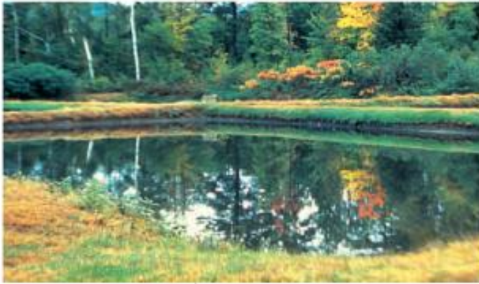
Figure 74. Wastewater lagoon (United States Environmental Protection Agency, 2004).
