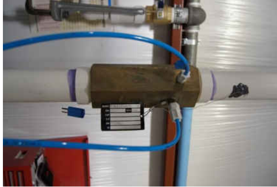
Figure 57: Venturi flow meter
