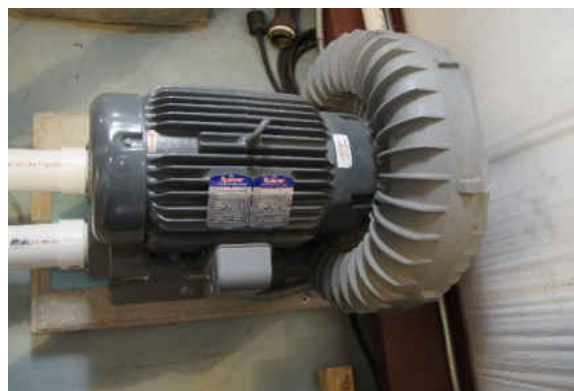
Figure 56: Regenerative vortex blower
