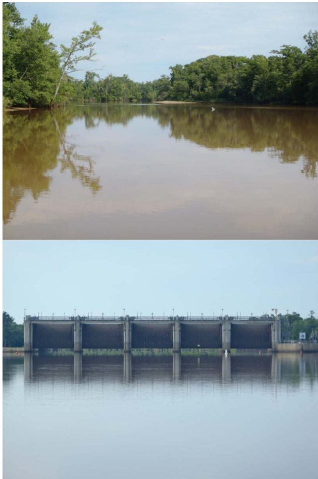
Figure 1. Top photo – Neches River channel upstream from the saltwater barrier; bottom photo – saltwater barrier on Lower Neches with gates in open position.
