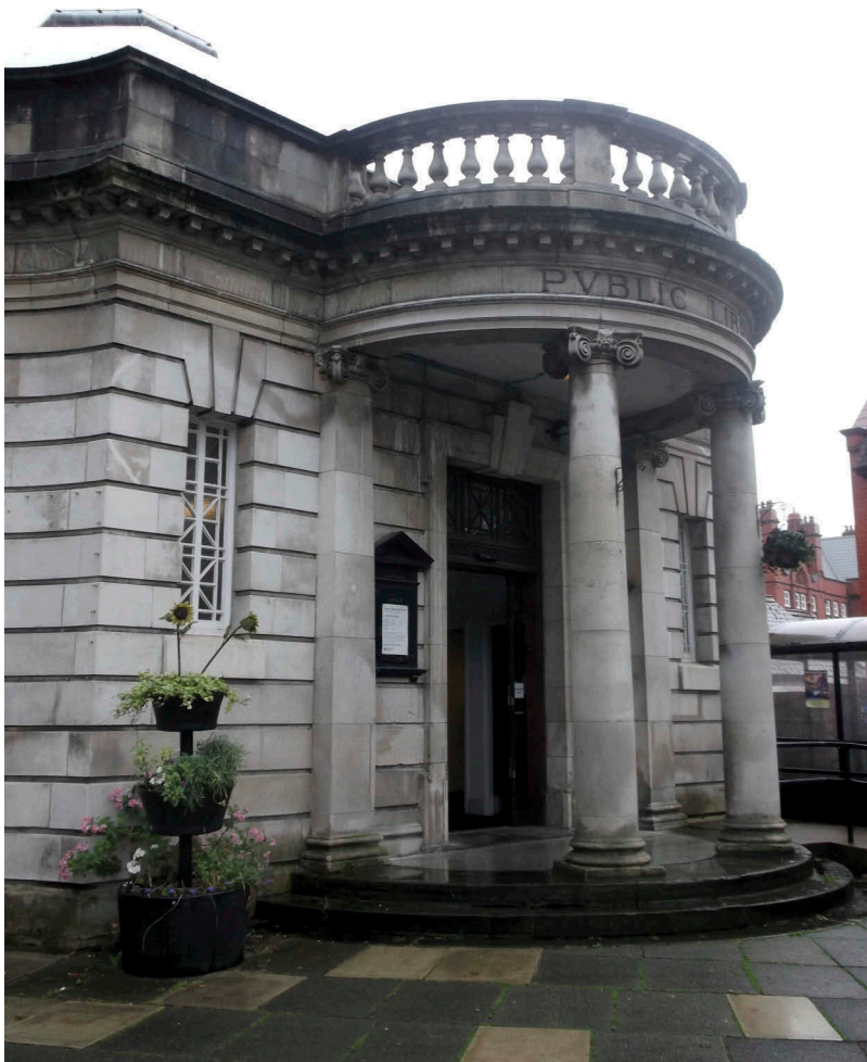
Figure 3. Library, photo by Fiona.
