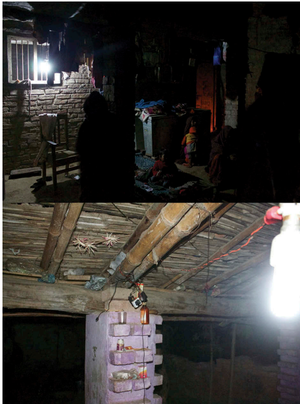
Figure 3. A lightbulb installed on the window to light multiple spaces (top). A bulb with plugs for charging mobile phones and spaces created for them (bottom). (Source: Author)
