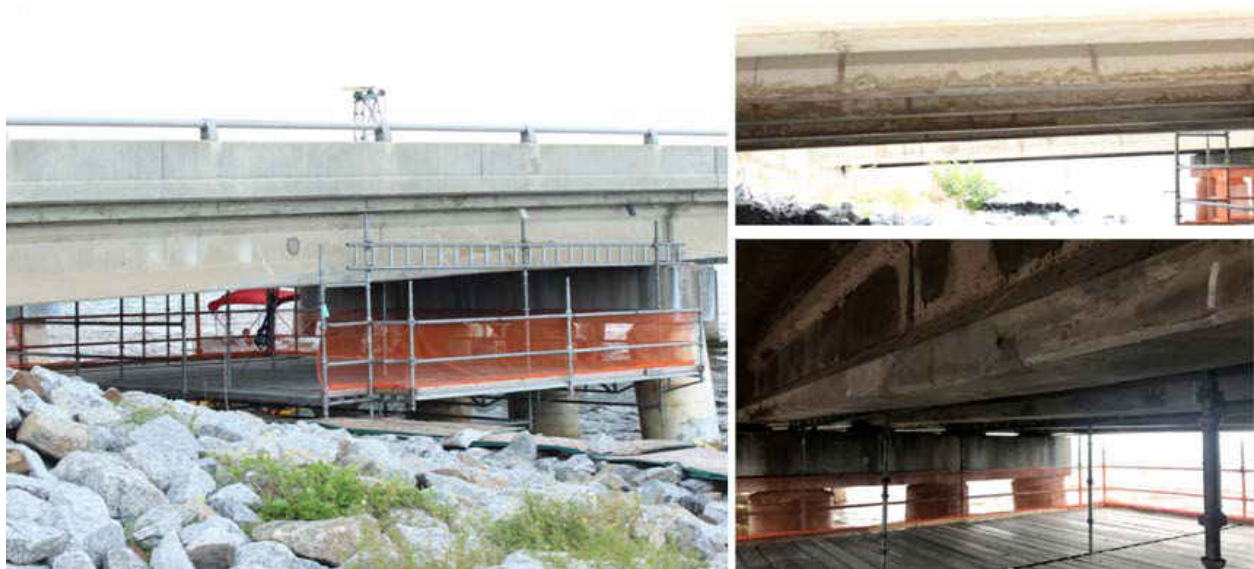
Figure 102 The prestressed concrete highway bridge in this study
