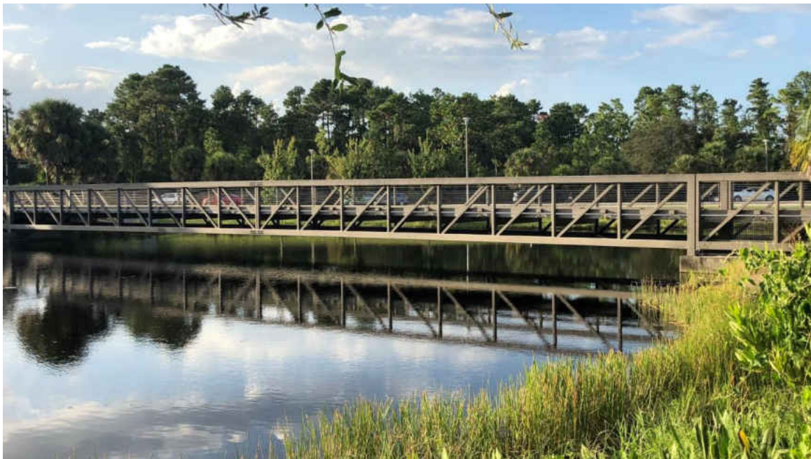
Figure 1.2: Parking Garage VI – H Pedestrian Bridge on UCF campus
