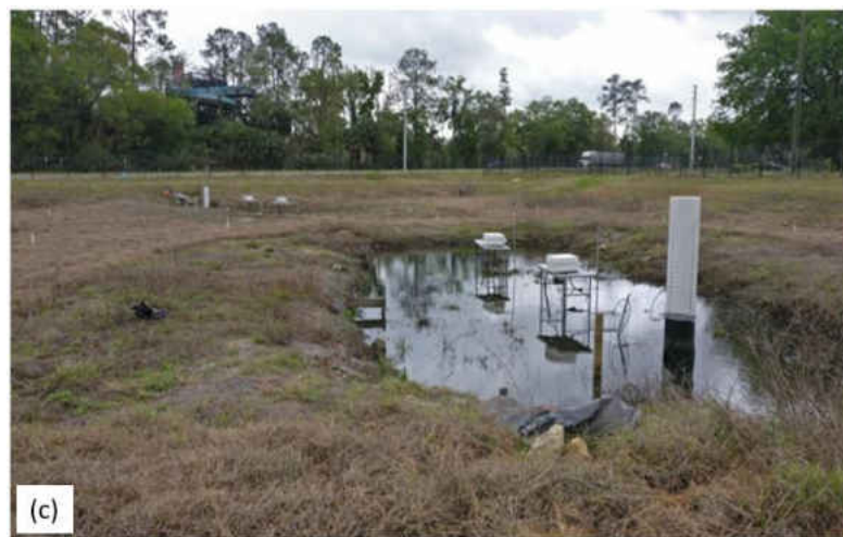
Figure 1: (a) Nitrate treatment through BAM blanket filter constructed in a stormwater retention basin. (b) The design concepts and general dimensions of blanket filters. (c) A constructed blanket filter in City of Ocala, Florida (Wen et al., 2019).
