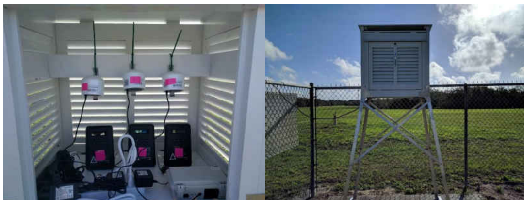
Figure 5-1. Pictures of sensor deployment (left: internal layout of the shelter; right: external appearance of the shelter).
