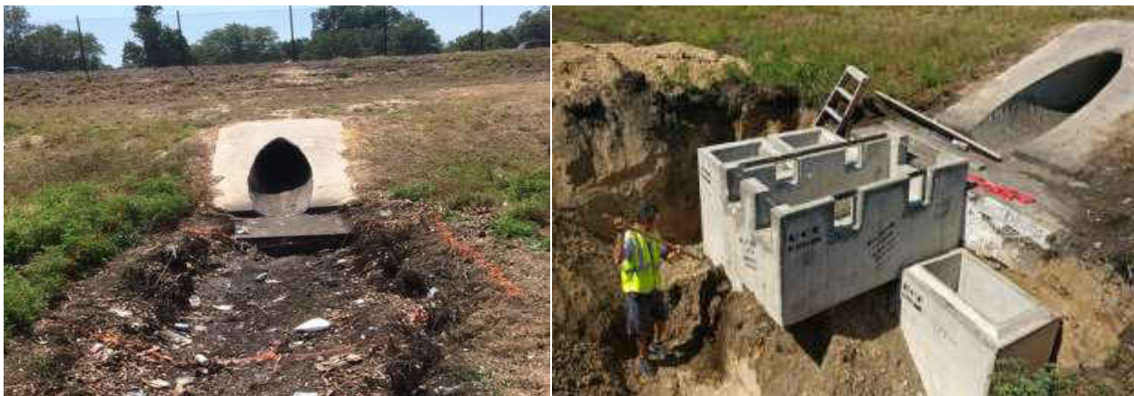
Figure 16: Construction of Vertical Reactors
