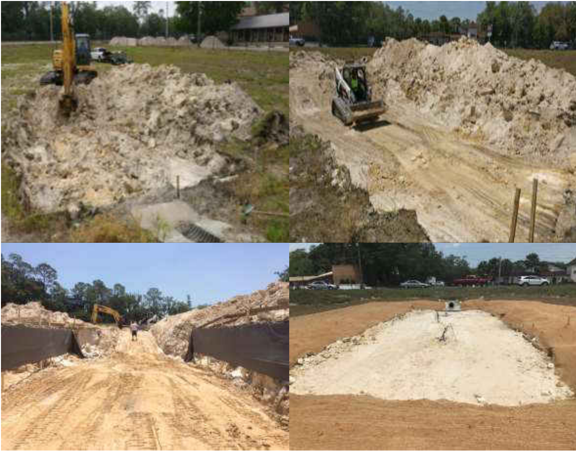
Figure 13: Construction of Blanket Filers
