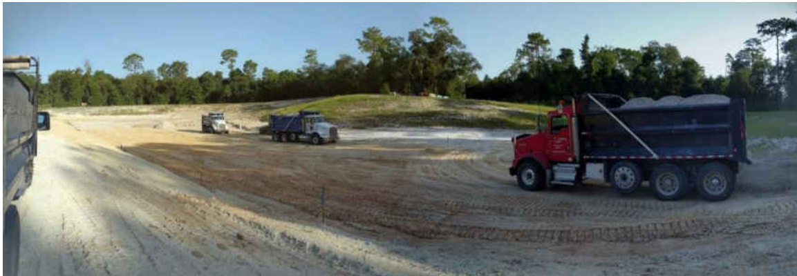
Figure 7. Installation of BAM in the Treatment Media Pond (July 2016)
