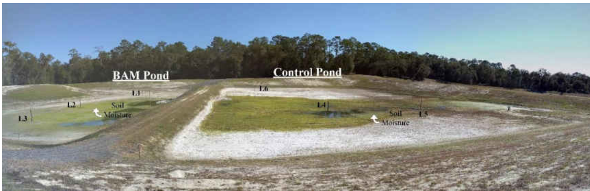
Figure 11. RIB Field Collection Layout and Water Puddling.
