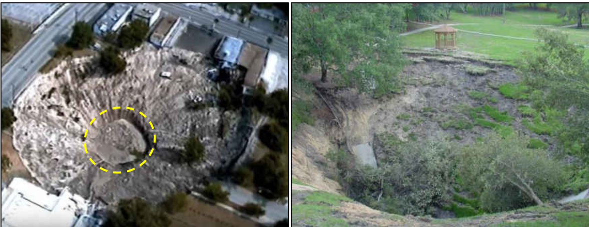
Figure 2-3: Photos of devastating cover collapse sinkholes in central Florida
