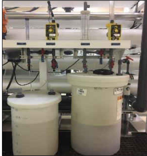
Figure 4-3: Scale Inhibitor Tank (left) and Sulfuric Acid Tank (right)
