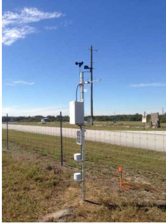
Figure 4-2 Fog Monitoring System (FMS) sensor
