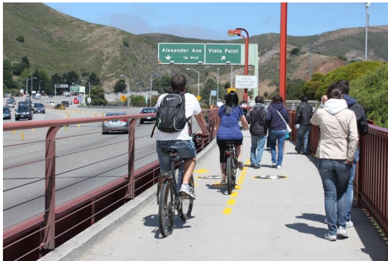
Figure 14. Pedestrian Sidewalk Barrier (source: goldengate.org)
