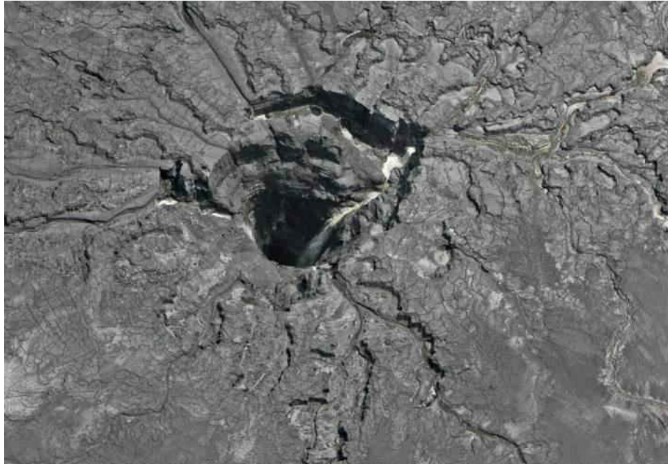
Figure 1. Aerial image of sinkhole occurred in Mulberry, FL (Tampa Bay Times, 2016)
