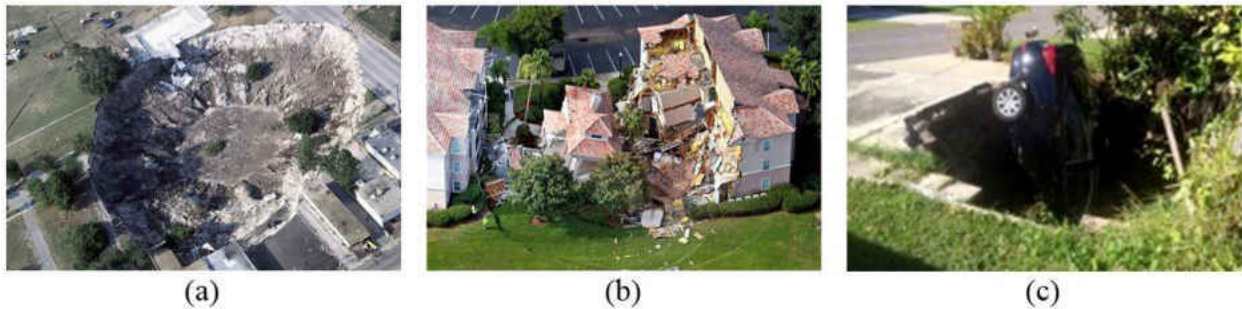
Figure 2. Cover-collapse sinkhole occurrences in Florida: (a) Winter Park, FL (1981), (b) Orlando, FL (2013), and (c) Pasco County, FL (2014)
