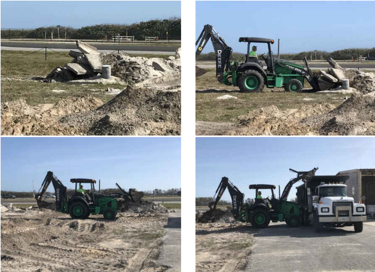
Figure 1: Hauling of concrete waste on Patrick Air Force Base, Florida
