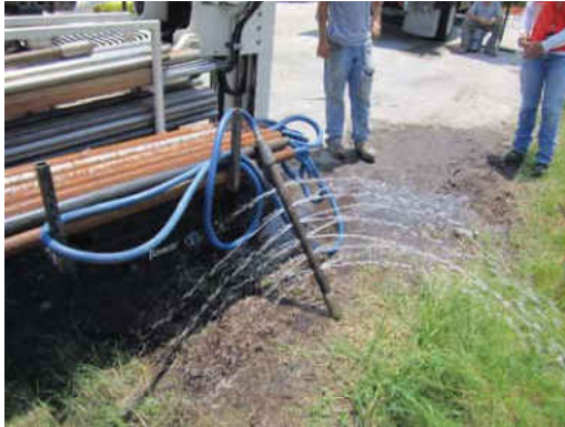
2 ft Injection tool during water test
