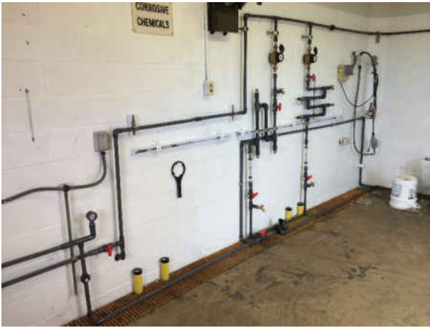
Figure 4-2: Manele Bay WWTF Corrosion Control Skid (a) Control rack (b) Test rack
