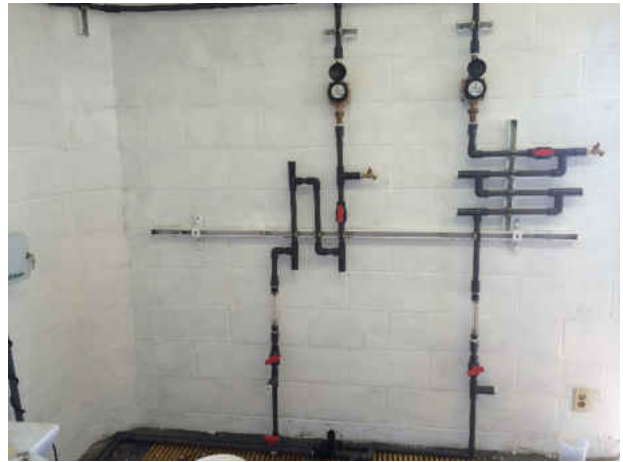
Figure 4-2: Manele Bay WWTF Corrosion Control Skid (a) Control rack (b) Test rack
