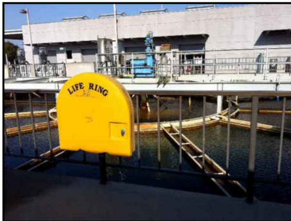
Figure A-4: Photo of the MSJWTP full-scale solid-contact clarifier
