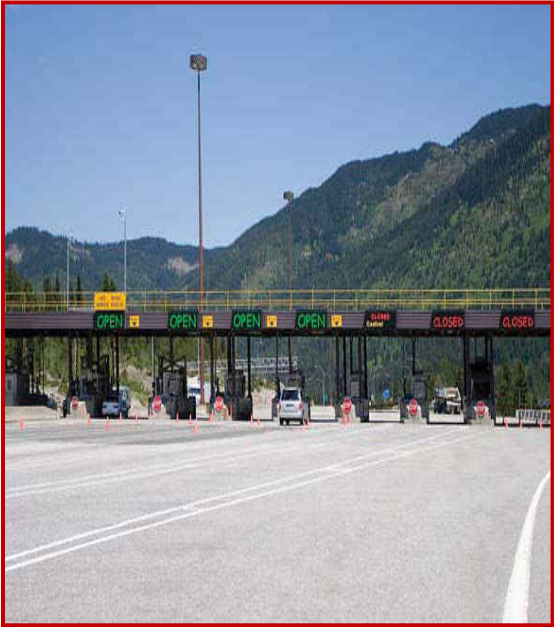
Figure 4-8: Traditional Mainline Toll Plaza (TMTP) (Source: FHWA, 2014)
