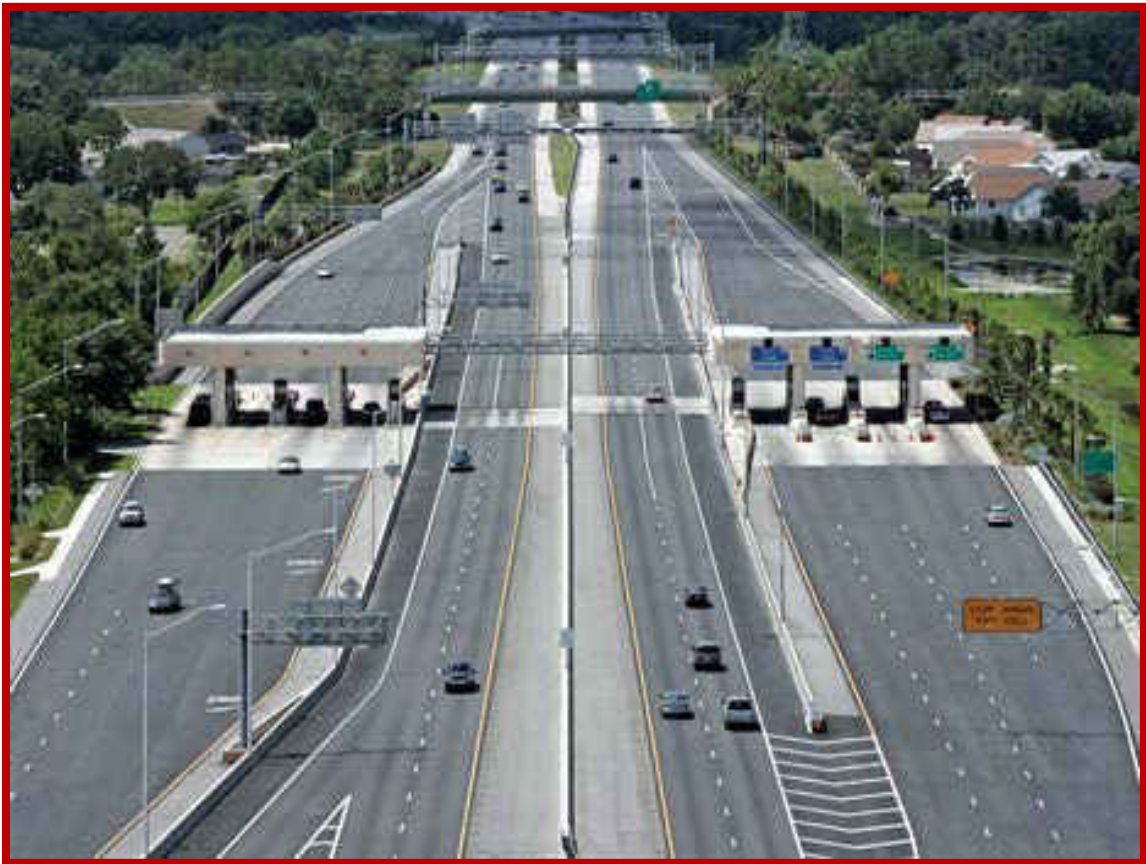
Figure 2-12: HTP the ORT in the mainline (Source: CFX, 2014)
