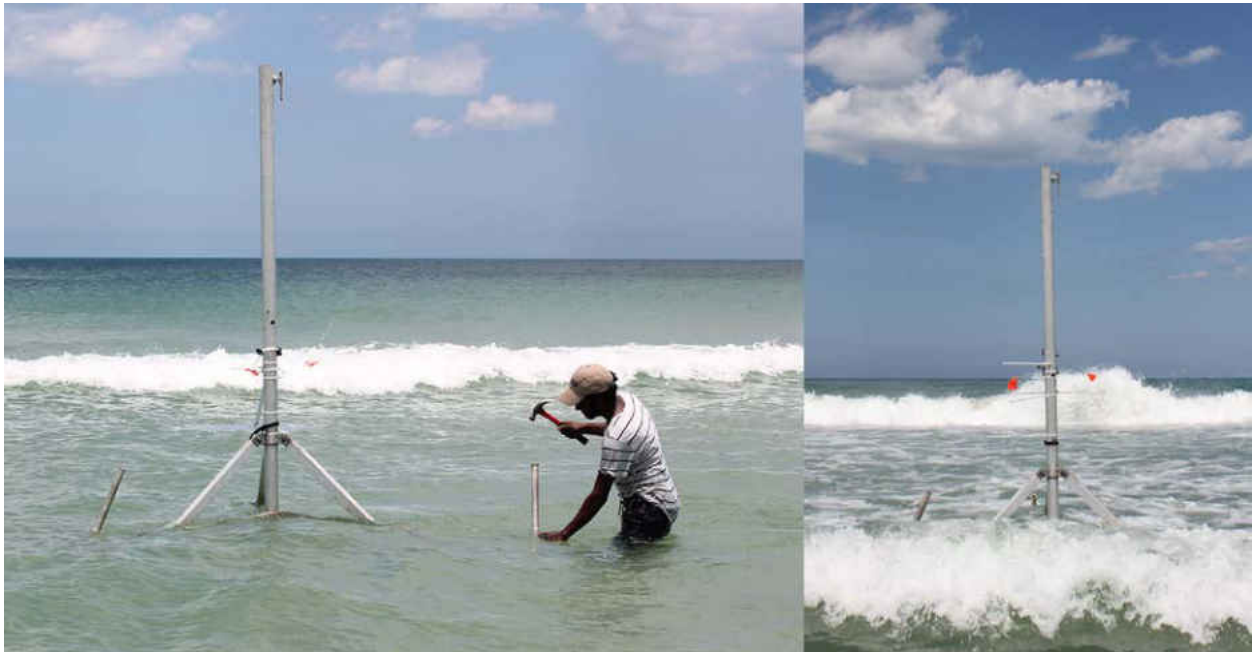
Figure 37: Project 2 securing rig in ocean and rig withstanding waves, By Author, 2016
