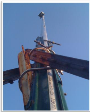
Figure 17: Anchoring structure of the relay pole.
