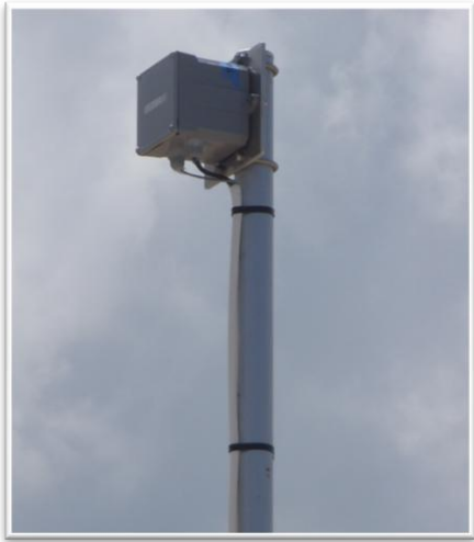
Figure 13: Directional transmitter on top of Turtle Cam array.
