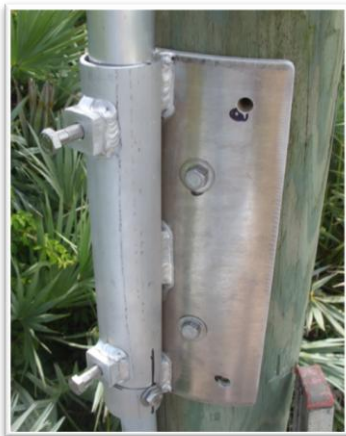
Figure 15: Original relay pole bracket.
