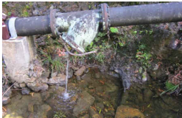
Figure D-3 Second Caisson Pipeline
