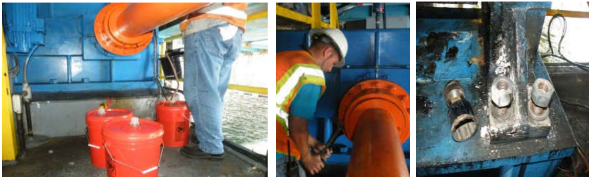
Extracting the Oil from the Gearbox
