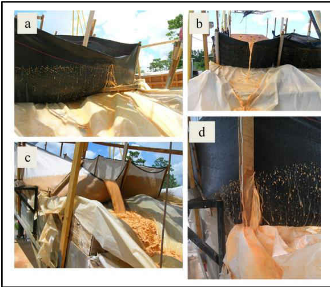
FIGURE 16 SILT FENCE FAILURES: (A) PULLOUT OF FABRIC FROM MIDDLE STAKE ON 33% SLOPE (B) OVERTOPPING ON 33% SLOPE (C) CORNER STAKE FAILURE ON 33% SLOPE (D) CORNER STAKE TEAR ON 25% SLOPE
