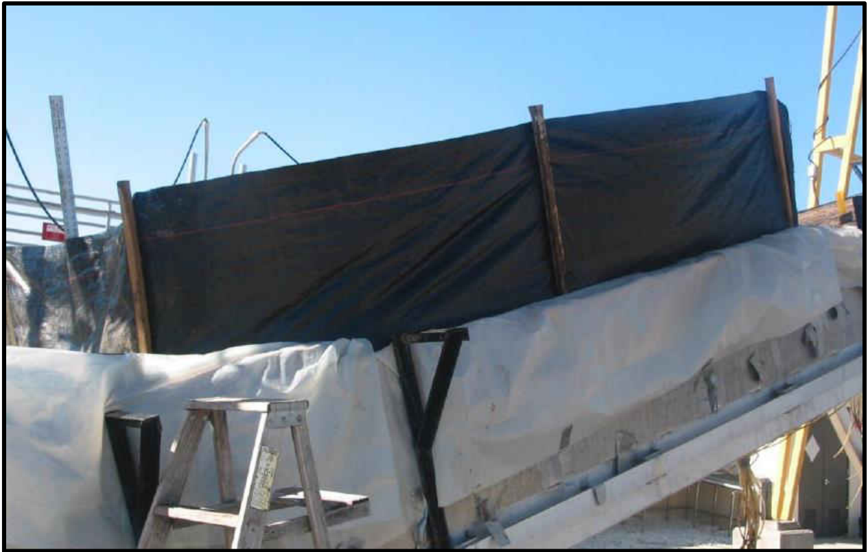
FIGURE 3 WOVEN (ASR 1400) SILT FENCE INSTALLED ON A TILTED TEST BED (GOGO-ABITE 2012)
