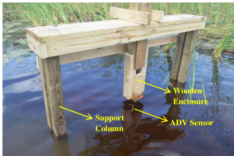
Figure 4.3: Sensor support structure
