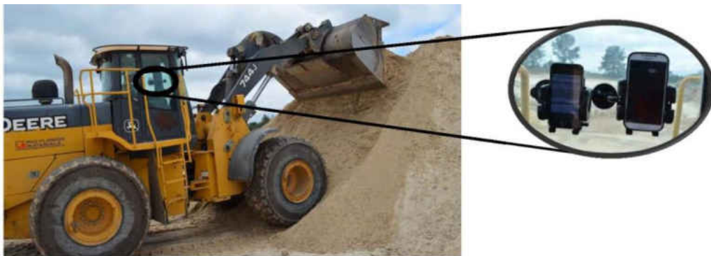
Figure 4.3: Smartphones mounted inside the front-end loader cabin.
