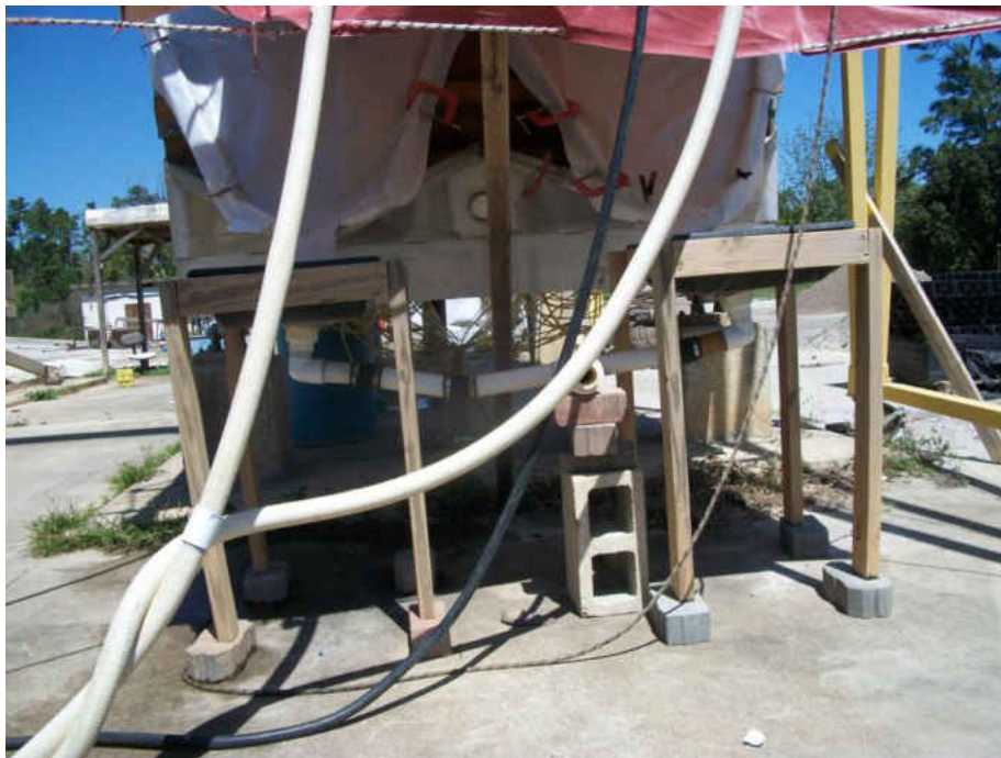
Figure 15: Downstream Collection Troughs and Sinks
