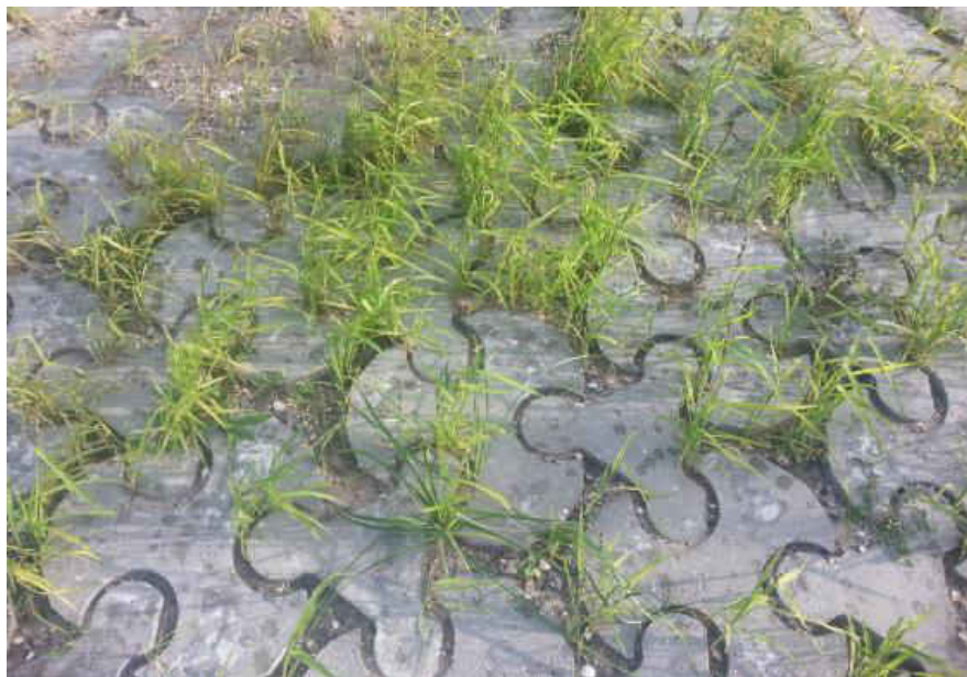
Figure 4-26 Vegetative regrowth between blocks approximately 2 months following installation.
