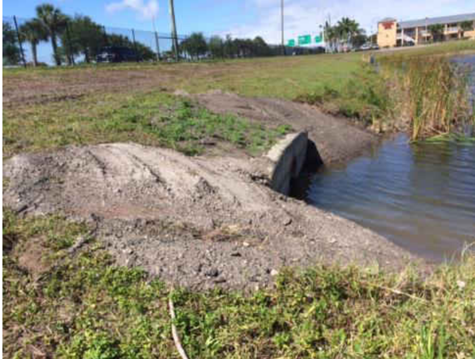
Figure 4-3 Inlet #2 shortly following re-filling of the bank, picture taken March 25 th , 2014.
