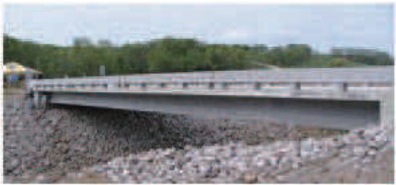
(b) The first UHPC bridge in U.S.: Wapello County Bridge ([25])
