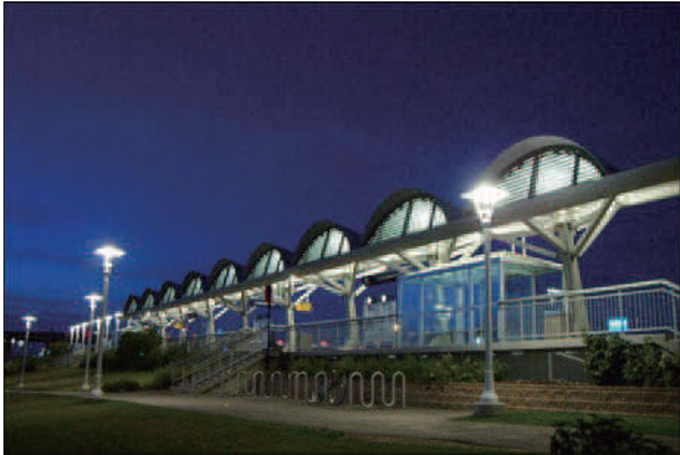
Figure 3: THE SHAWNESSY LIGHT RAIL TRANSIT STATION PHOTO 1
