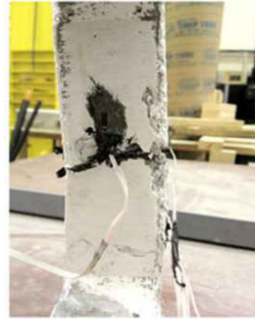
Strain Gage failure Closeview
