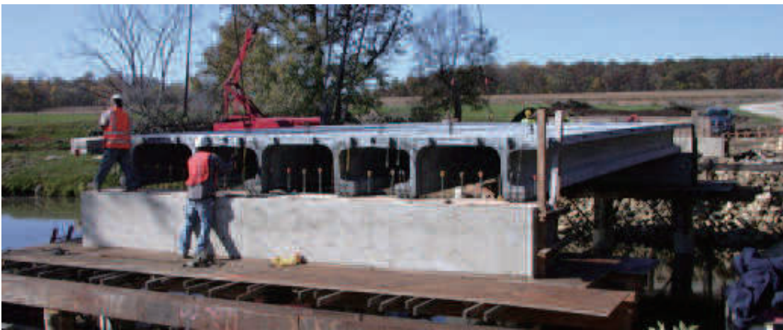
Figure 5: THE JAKWAY PARK BRIDGE PHOTO 1
