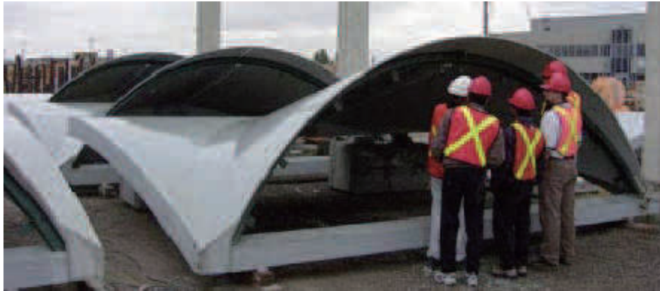
Figure 4: THE SHAWNESSY LIGHT RAIL TRANSIT STATION PHOTO 2
