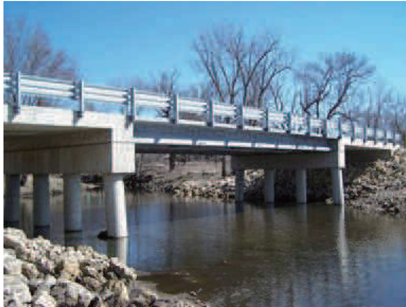
Figure 6: THE JAKWAY PARK BRIDGE PHOTO 2
