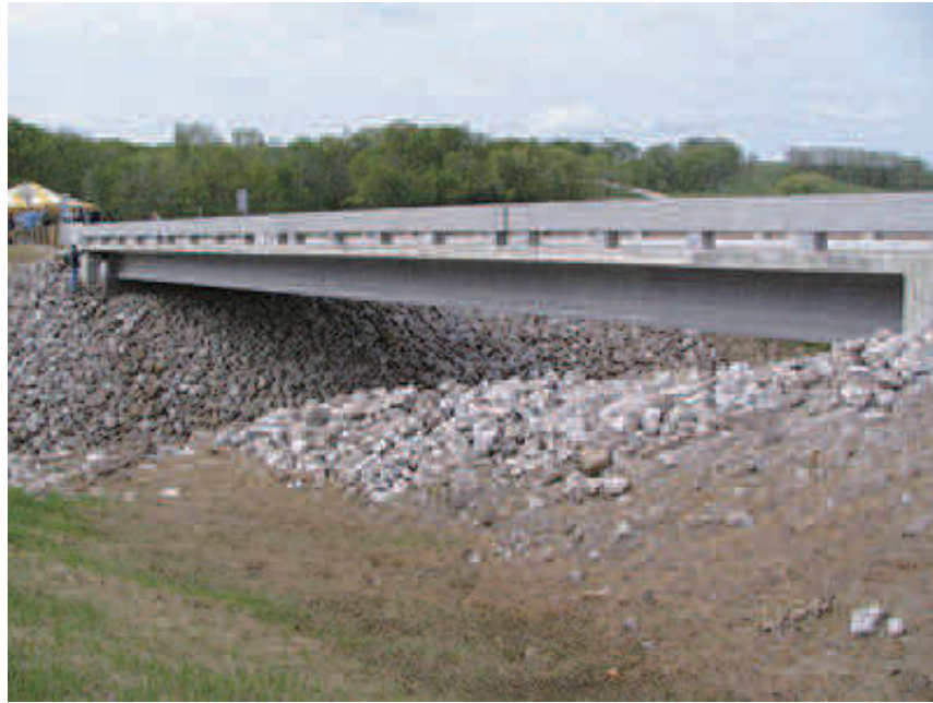
Figure 7: MARS HILL BRIDGE IN WAPELLO COUNTY PHOTO 1
