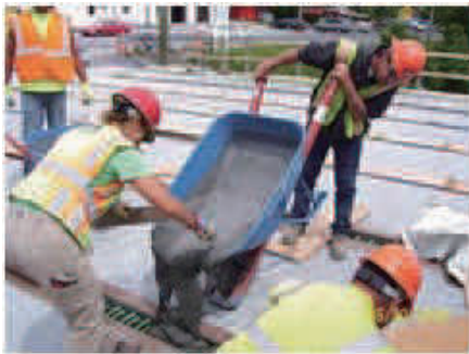
(a) Longitudinal connections cast between deck-bulb-tee girders ([25])
