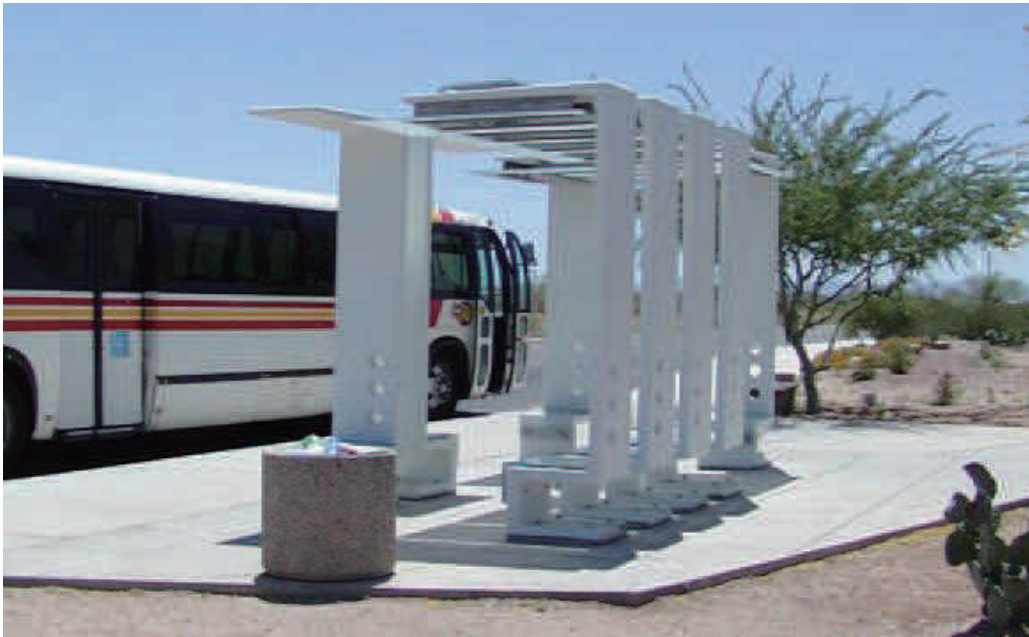
Figure 9: BUS SHELTERS MADE OF UHPC
