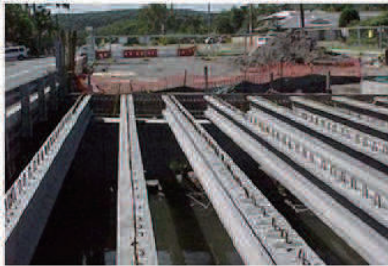
Figure 11: THE SHEPHERDS CREEK DUCTAL BRIDGE PHOTO 1
