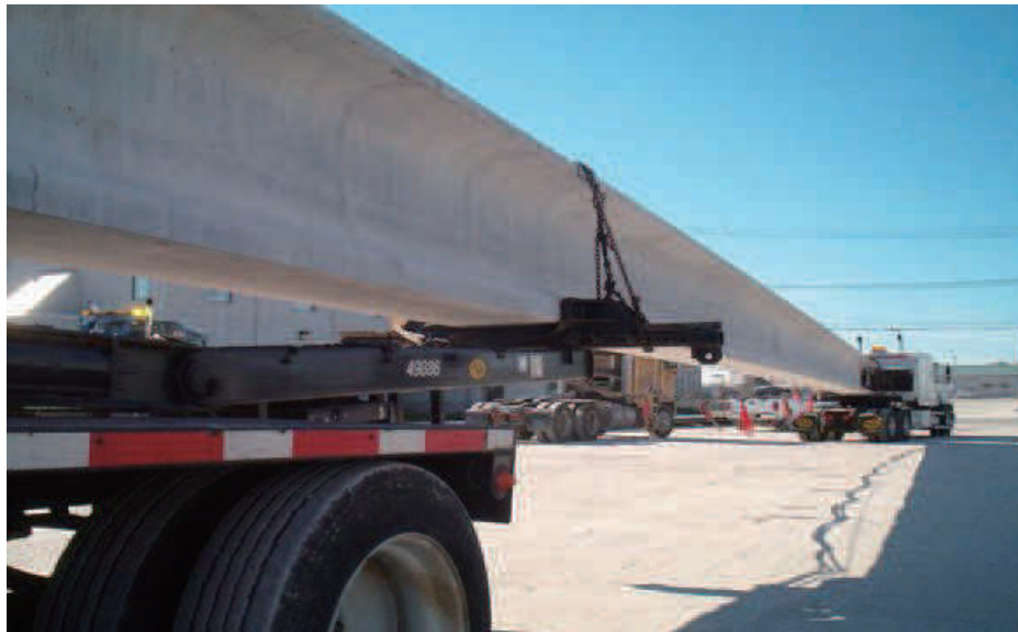
Figure 8: MARS HILL BRIDGE IN WAPELLO COUNTY PHOTO 2
