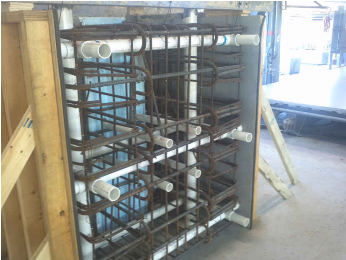
Figure C.12: Reaction Block at Gate Precast Company Prior to Pour
