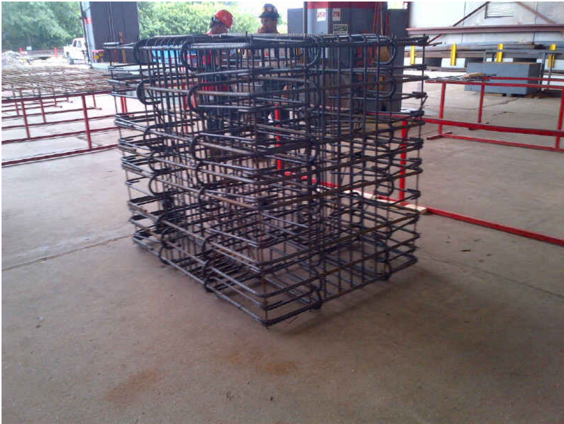
Figure C.11: Reaction Block at Gate Precast Company Prior to Pour
