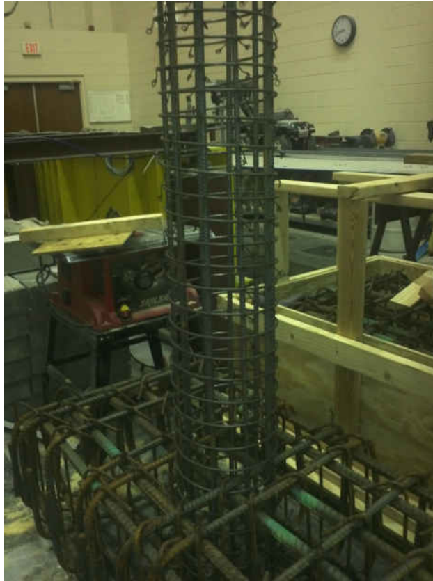
Figure 3.11: Photo of Column Reinforcing
