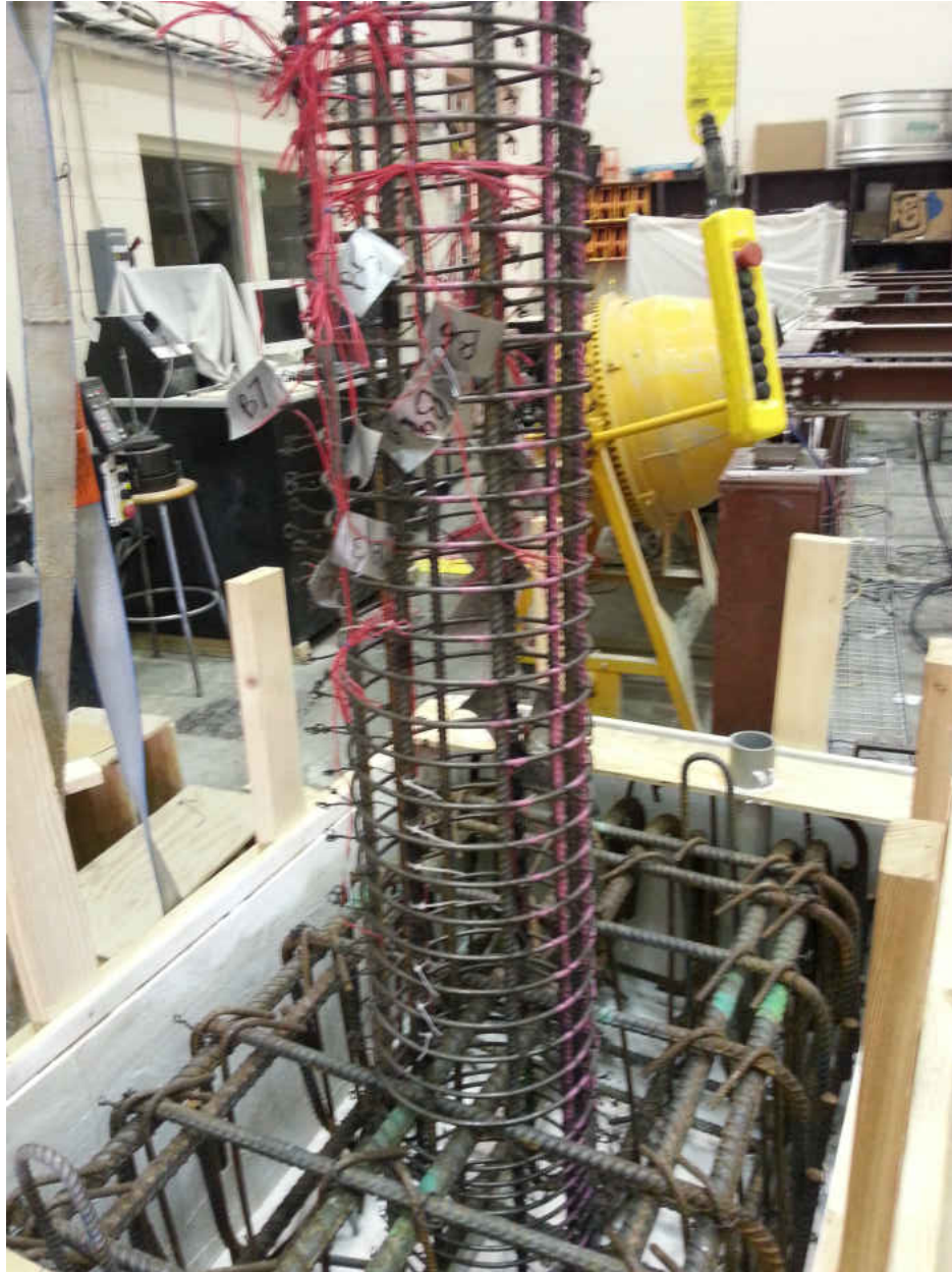
Figure C.1: Column Photo Prior to Pour
