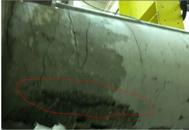
Figure 4.34: Photo Showing Longitudinal Reinforcing Bar Buckling from the Damage Phase
