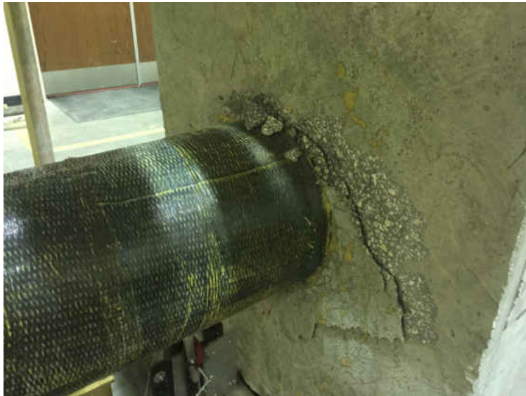
Figure 4.38: Post-Repair Typical Column Failure
