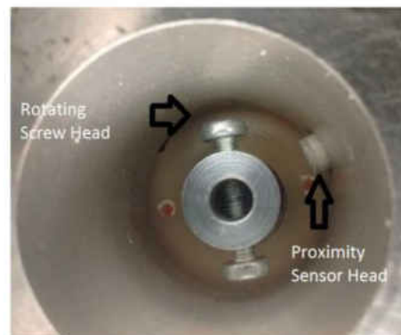
Figure 24 – Proximity Sensor installation [1]
