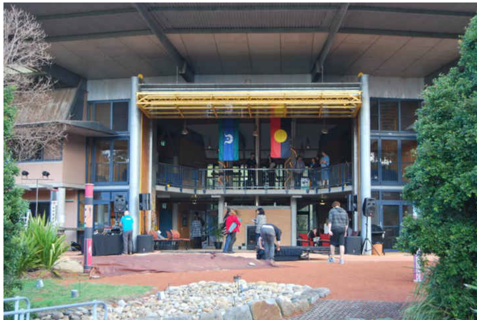
Figure 43. Glass wall open in preparation for an indoor/outdoor event at Sweet Grass.
