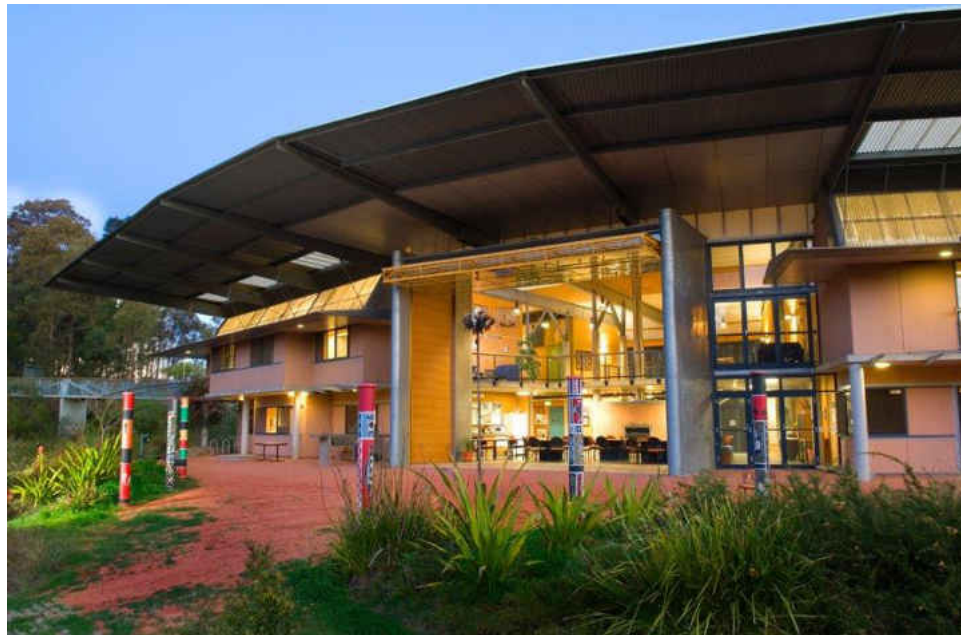
Figure 25. The Birabahn Building where Sweet Grass is housed.
