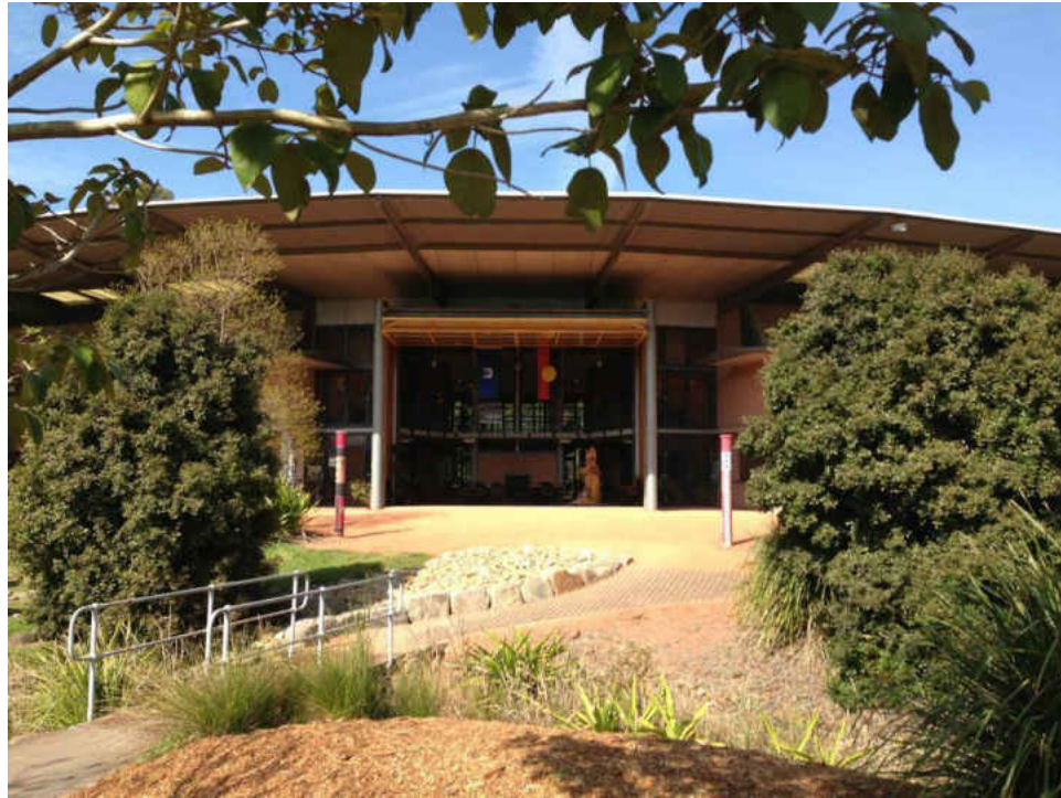
Figure 42. Entrance of Sweet Grass with glass wall that is open.
