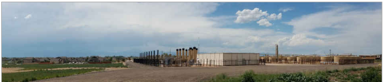
Figure 3. Large multi-well oil and gas production facility near residential subdivisions in the Town of Mead in Weld County, Colorado (Photo by the author)
