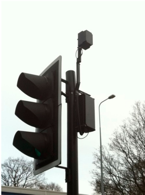
Figure 4. Typical Bluetooth installed on a traffic signal pole.
