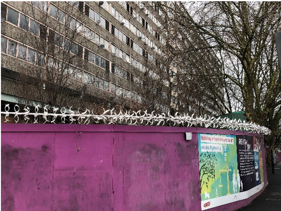
Figure 3. Aylesbury Estate's 'Alcatraz fence' built by Southwark Council around Chiltern House (Photo: Loretta Lees, 2018).
