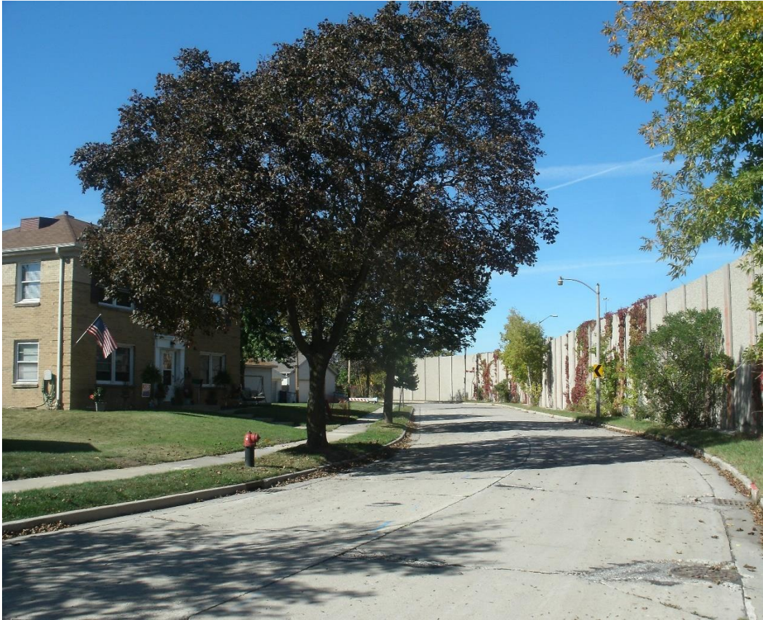
Figure 7: A concrete sound barrier separates I-43 from a residential neighborhood near South 5 th Street and West Warnimont Avenue. Photo by Greg Dickenson, 2013.
