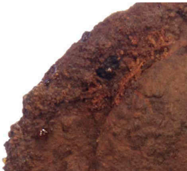
Figure 29. The hardened “rust bubbles” are what is left behind after post-excavation chloride weeping.
