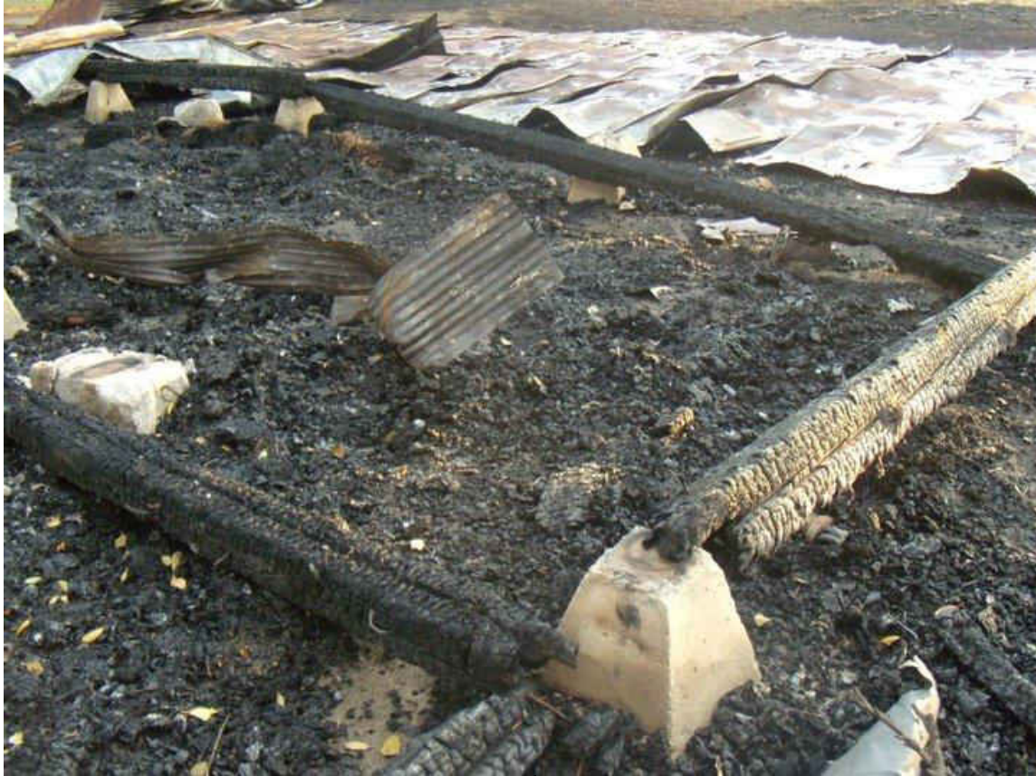
Figure 48. Photograph showing an Early 20 th Century out building constructed of beam over pilings support. Burnt 7/22/11 in Register, GA. View #2
