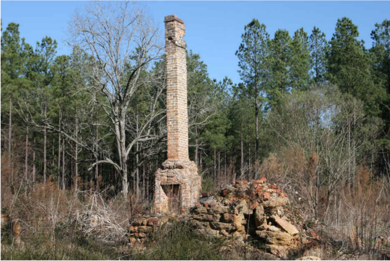
Figure 40. Photograph of an example of a Standing hearth/chimney at Old Town Plantation in Jefferson County, GA (View #1)
