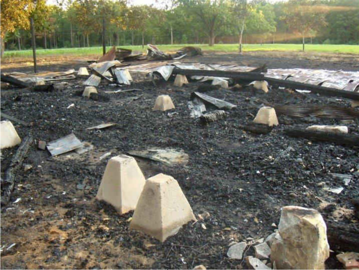
Figure 49. Photograph showing Early 20 th Century out building constructed of beam over pilings support. Burnt 7/22/11 in Register, GA. View #3
