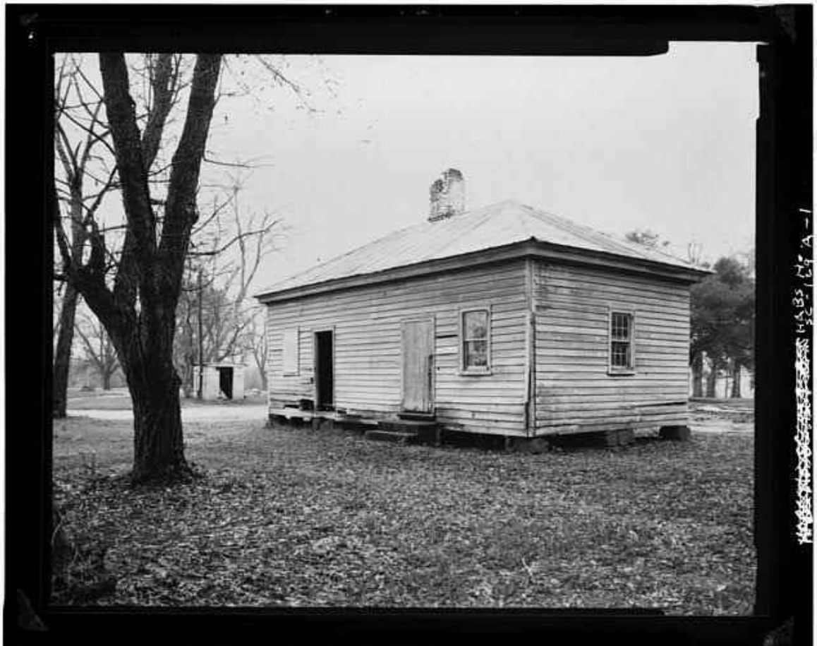
Figure 6. Photograph of Kensington Plantation, Summer Kitchen, U.S. Route 601, Eastover vicinity, Richland, SC. Exterior View (HABS SC,40-EAST.V,1A-1, 1982)
