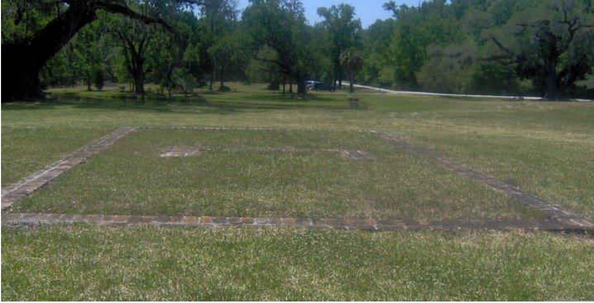
Figure 3. Photograph of brick foundation and hearth of Kitchen Structure at Drayton Hall, view from rear of house
