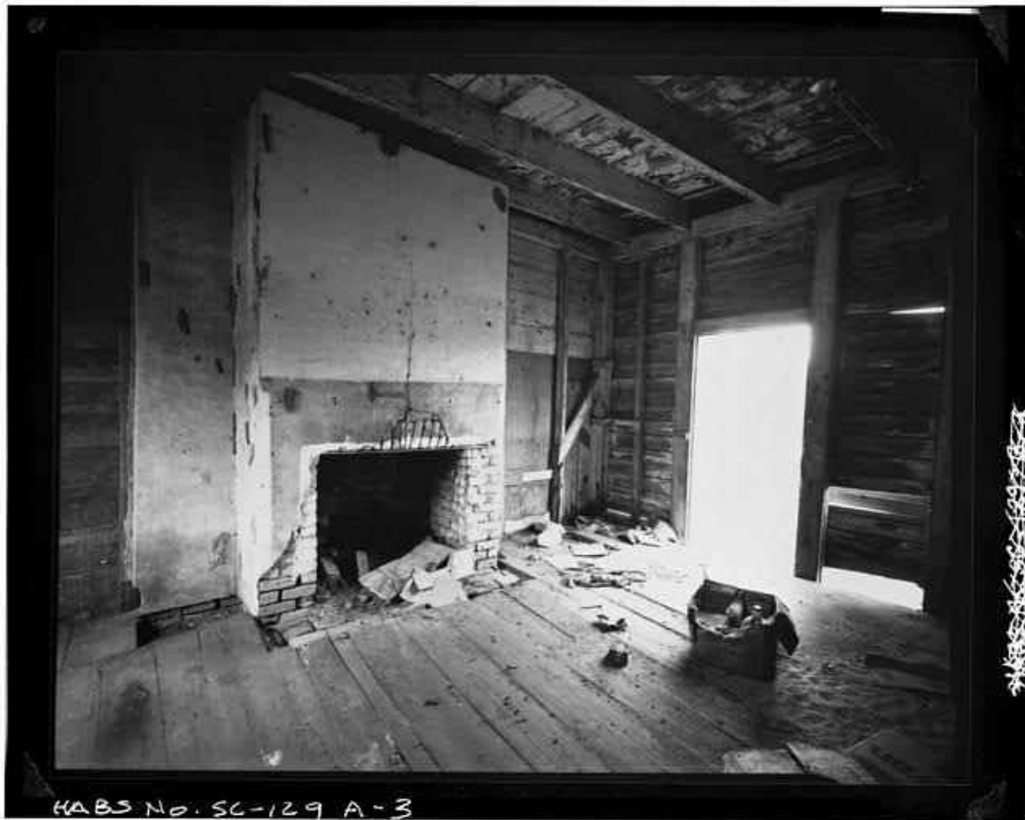
Figure 7. Photograph of Kensington Plantation, Summer Kitchen, U.S. Route 601, Eastover vicinity, Richland, SC. Interior View of Hearth (HABS SC,40-EAST.V,1A-3, 1982)
