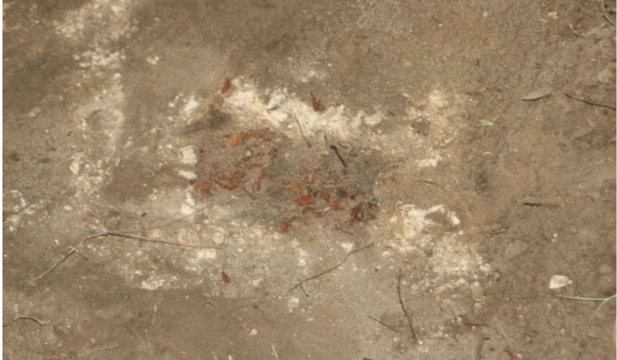
Figure 13: Third post in mortar.
