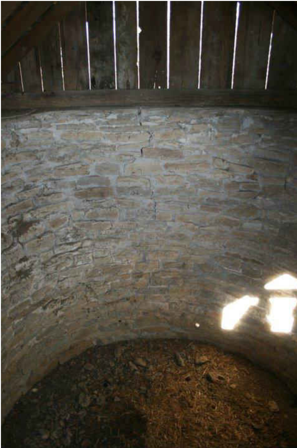
Figure 11. Ice house at Cassius M. Clay's plantation in Kentucky. Note the dirt floor. It is a circular ice house. Picture courtesy Misty Dunn.
