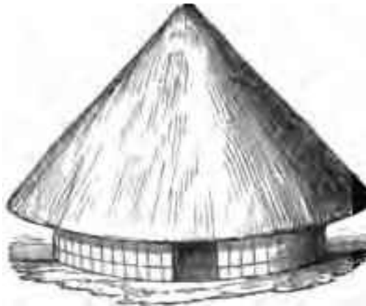
Figure 1. Conical shaped ice house with thatched roof.
