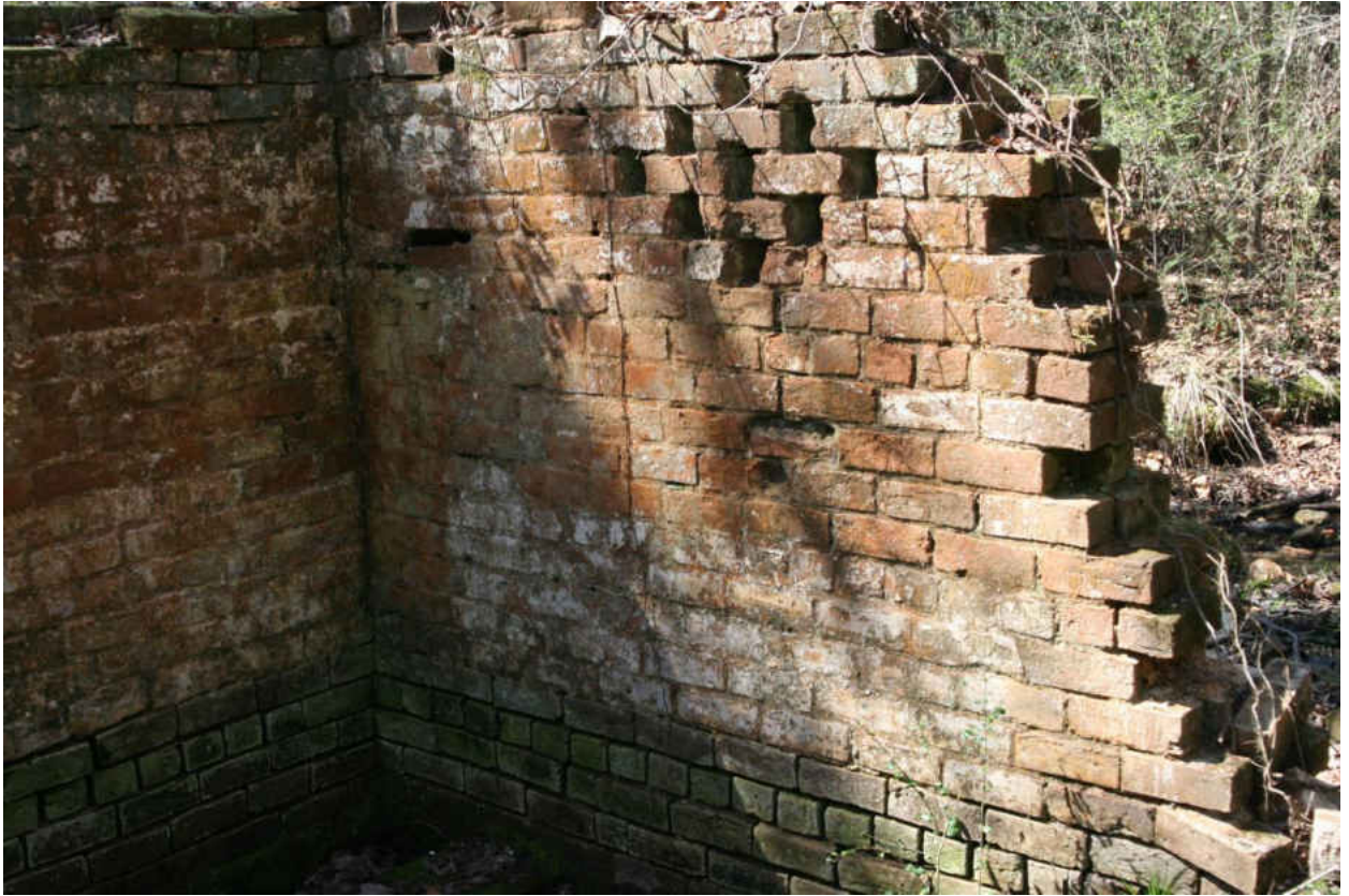
Figure 48. The springhouse at Old Town.
