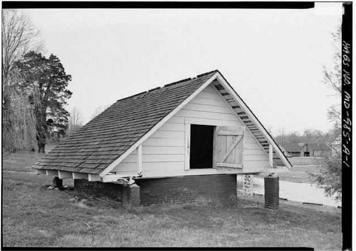
Figure 4. The Cottage, Ice House, Upper Marlboro, Prince George's Maryland. Perspective view looking Northwest. HABS MD, 17-MARBU,13A-1 Photographer Jack E. Boucher, 1990.
