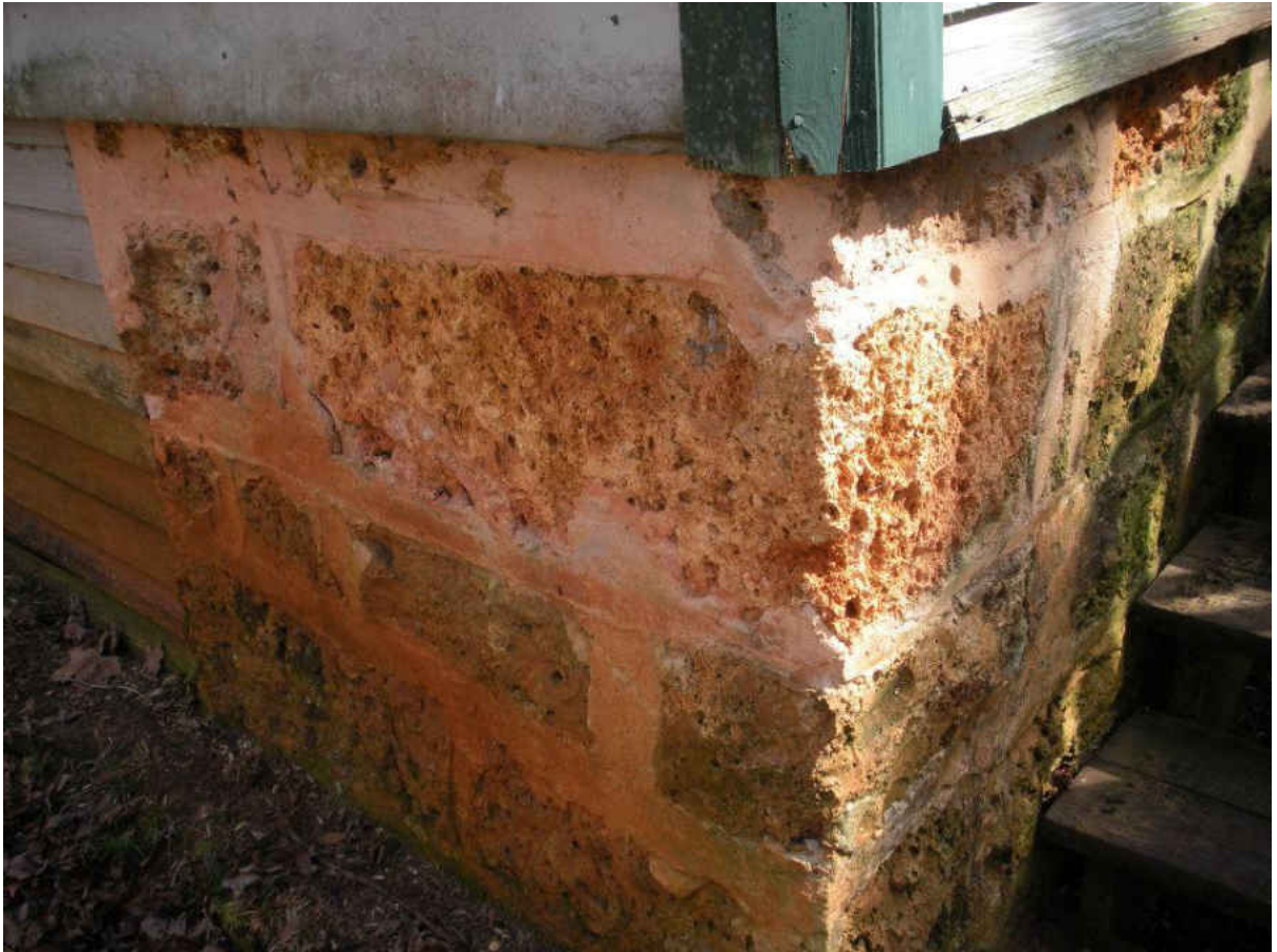
Figure 50. More of the chert that was found on the property and used for the foundation of the saw mill.
