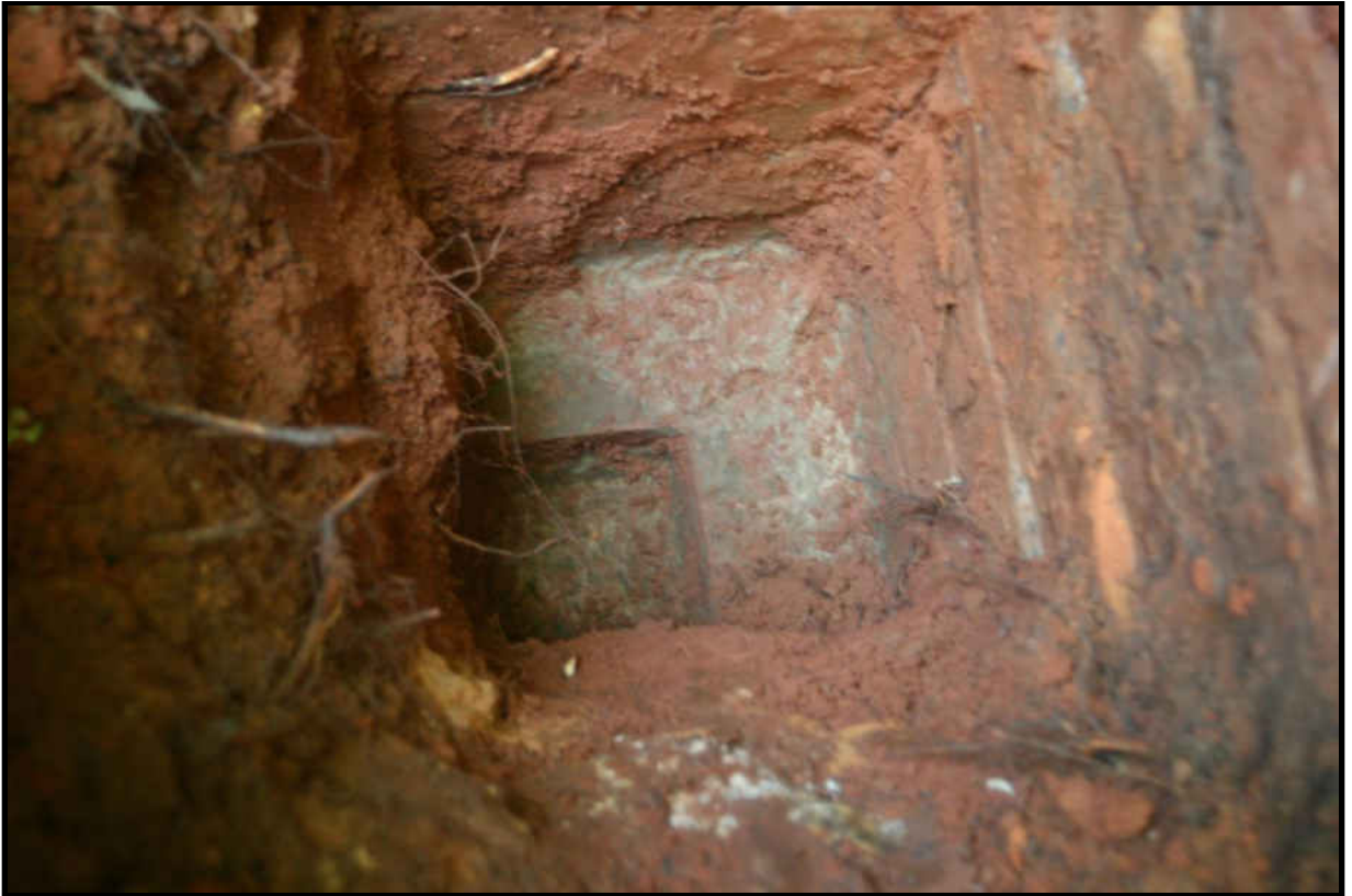
Figure 32. Photograph shows the ledge that runs around the bottom.
