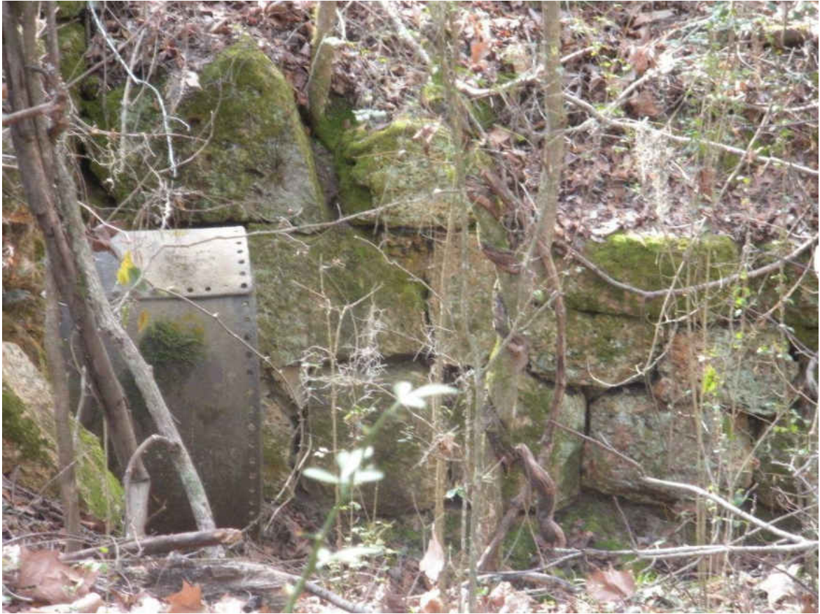
Figure 52. Chert found on the property and used to shore up the banks of the creek running to the saw mill.
