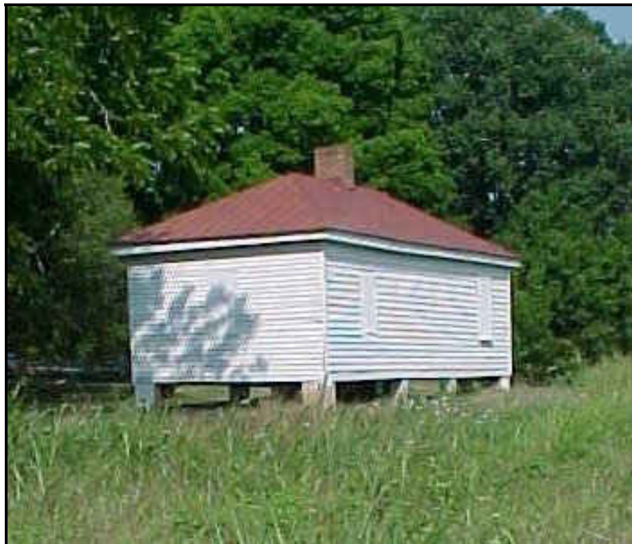
Figure 4.10: Photograph of Two-room Slave Quarters at Redcliffe Plantation, Aiken County, South Carolina.
