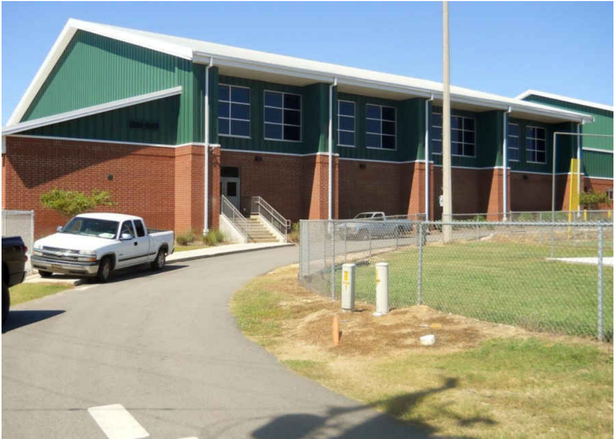
Rear entrance to Portal Middle High School Gymnasium.
