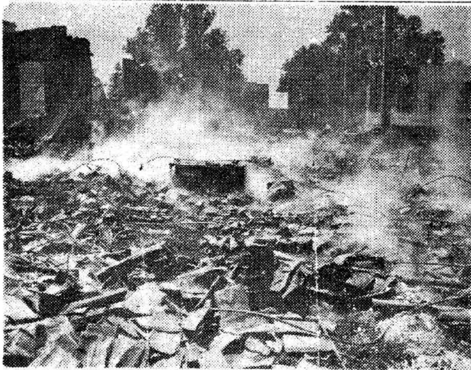
THIS WAS THE PORTAL SCHOOL —The smoking embers and debris above are all that is left of the fine school plant at Portal in Bulloch county. This is the high school building which with its contents was a total loss. The grammar school building was badly damaged at a total loss estimated at $75,000. The blaze started early Thursday morning. (Photo by L. B. Jones Studio, Statesboro.)
