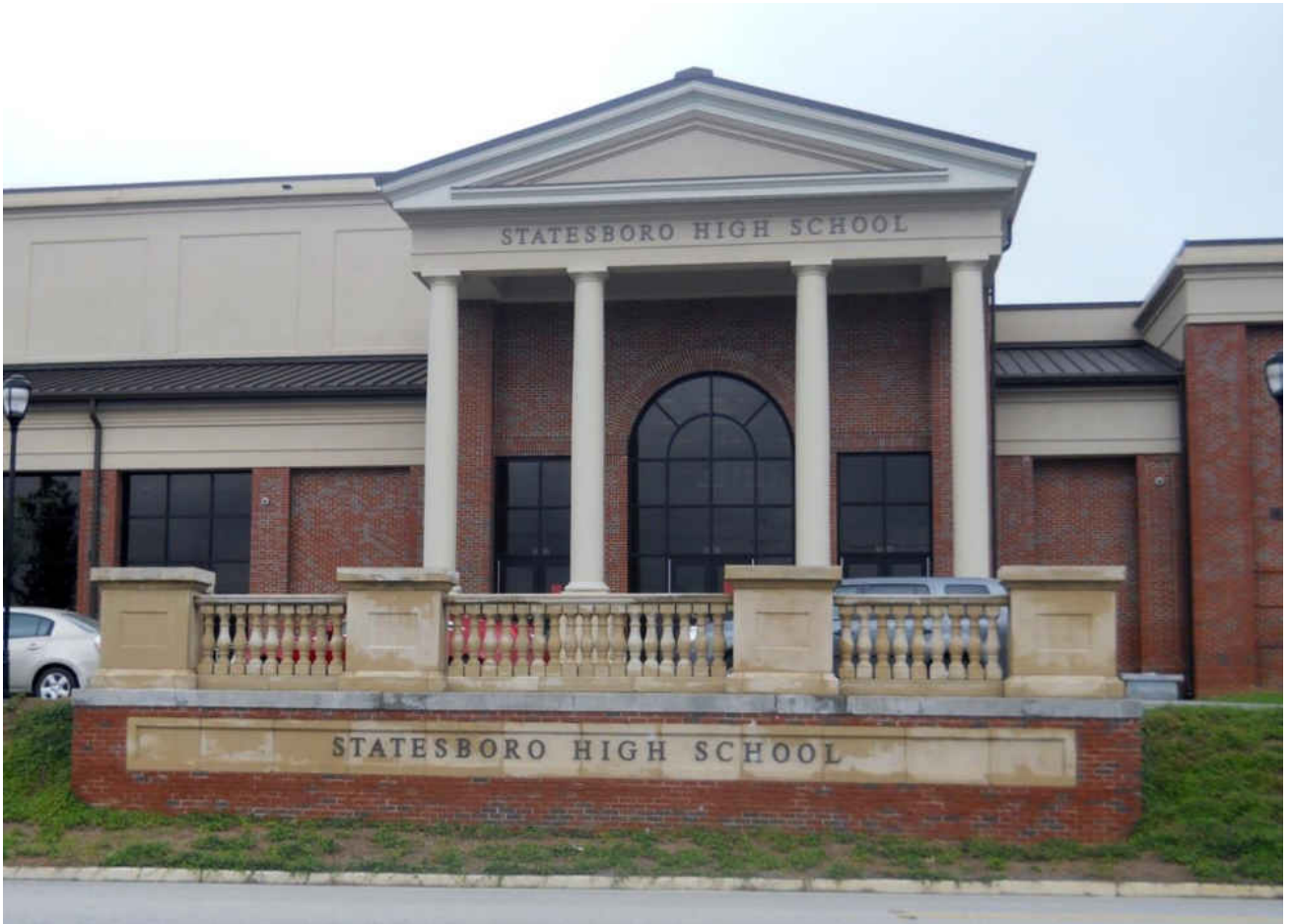
Front view of Statesboro High School as seen from Lester Road
