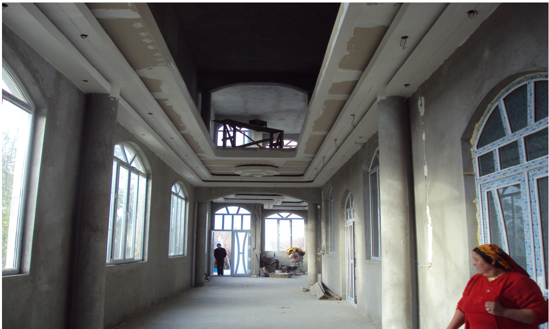
Figure 19 Liveni Caldadar house interior, unfinished construction . Photo taken by the author, 2010.
