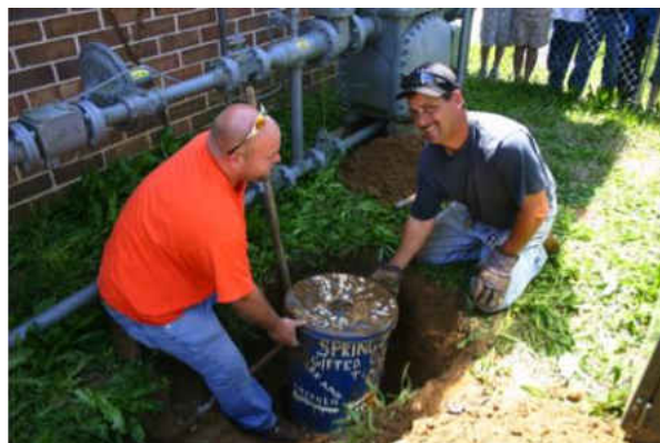
Figure 4. Workers remove capsule from the ground
