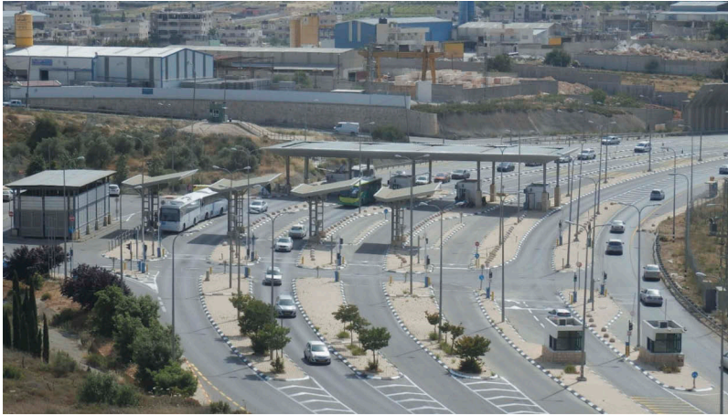
Figure 1. The tunnels checkpoint (source: photo by the author, May 2017).
