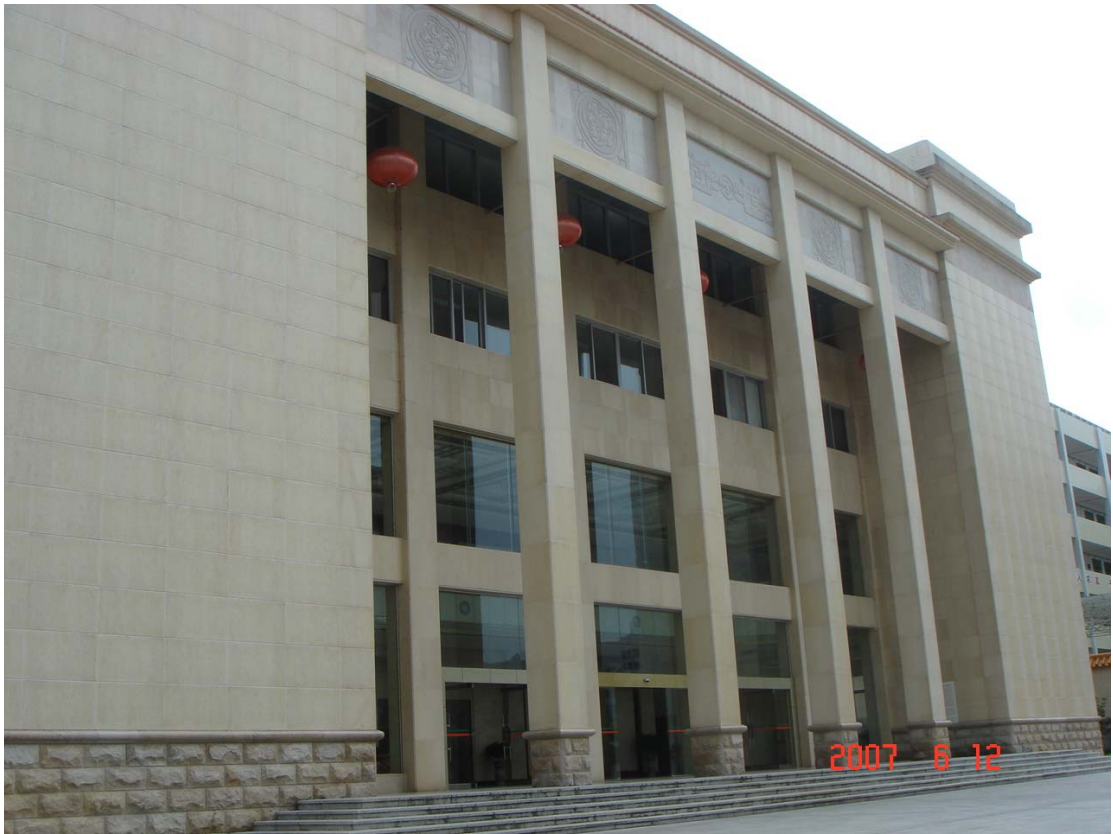
Picture 6.1 The new office building of the Dapu town government
