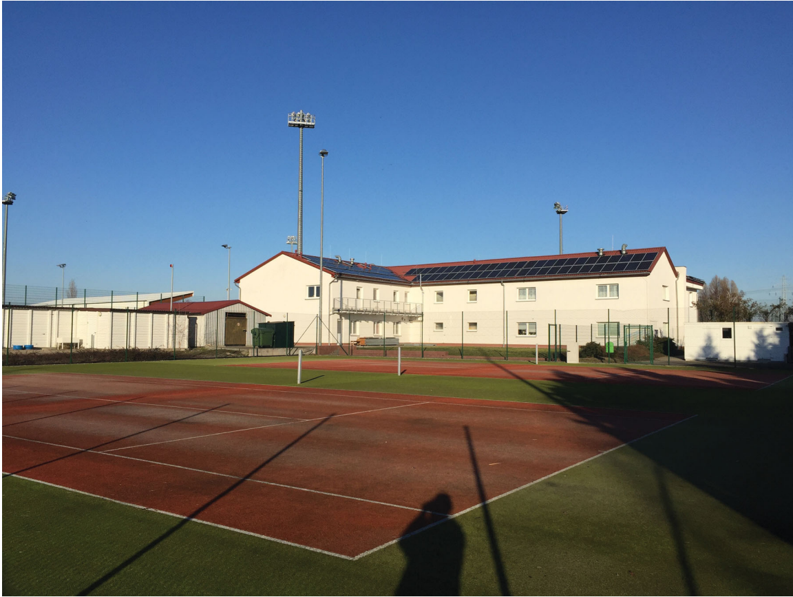
Figure 2. A sports club funded by Q Cells in Thalheim, complete with solar panels and floodlighting.
