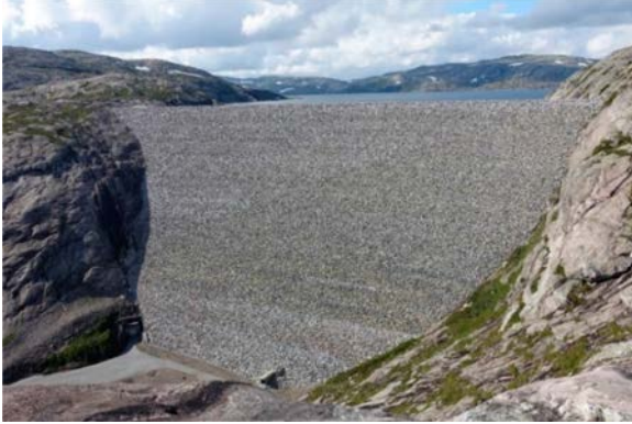
Figure 1. Downstream face of dam Svartevatn, Norway, built with narrow-steep abutment profiles (Photo P.H. Hiller, NTNU).
